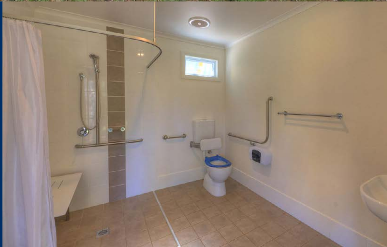
NEW DISABLED BATHROOM, Yea Riverside Caravan Park
